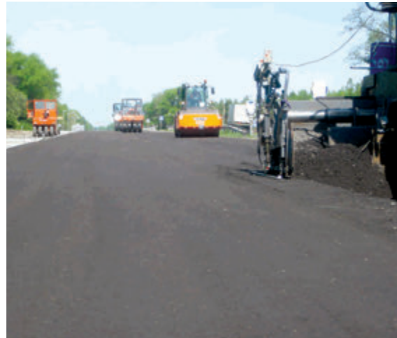
Cold Recycle Temel Serimi / Cold Recycle Base Paving
