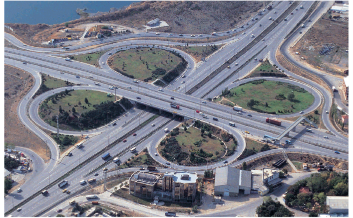
D 100 Devlet Yolu Kartal Kavşağı-İstanbul / D 100 Motorway Kartal Interchange-Istanbul
