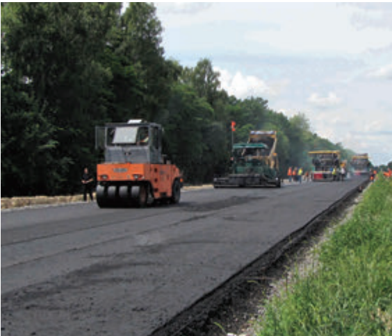
Kiev-Chop km 128-182 Otoyolu Yapım İşi / Kiev-Chop km 128-182 Highway Construction Project
